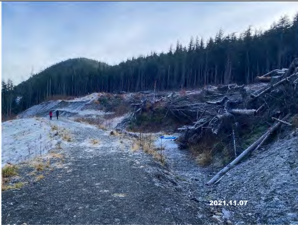
Partially Cleared Portion of Parcel
